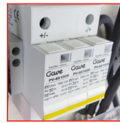
Surge protectors Phase connection on top and earth connection on bottom. Module end of life visual indication
