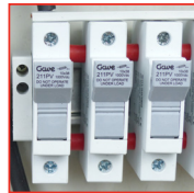
Fuse protection Positive and negative poles protected against overcurrents by gPV fuses
